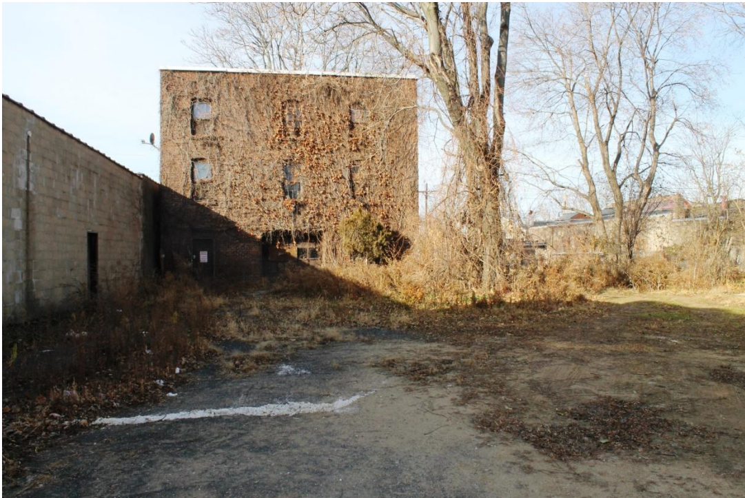
14 Myers Alley – Present Condition
